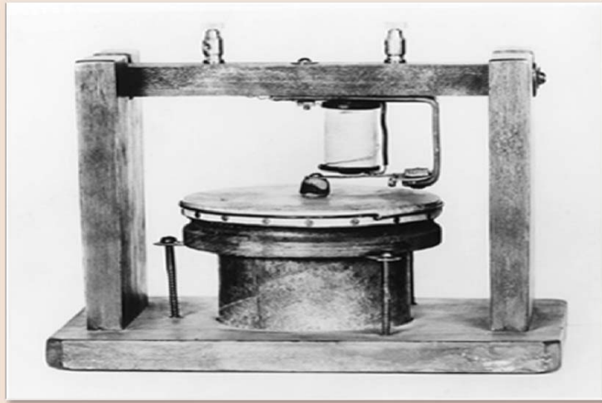
The first "Telephone"
