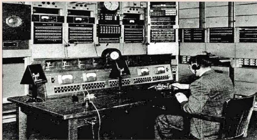
Typical AT&T network switch center (Washington) Bell Systems Technical Journal
