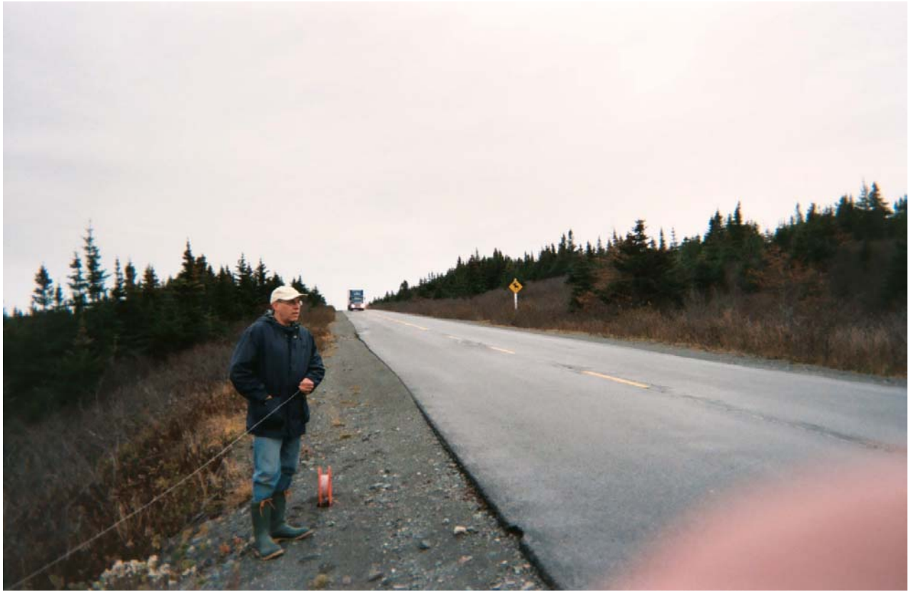
Here's Jean running wire along the road, trying to aim south.
