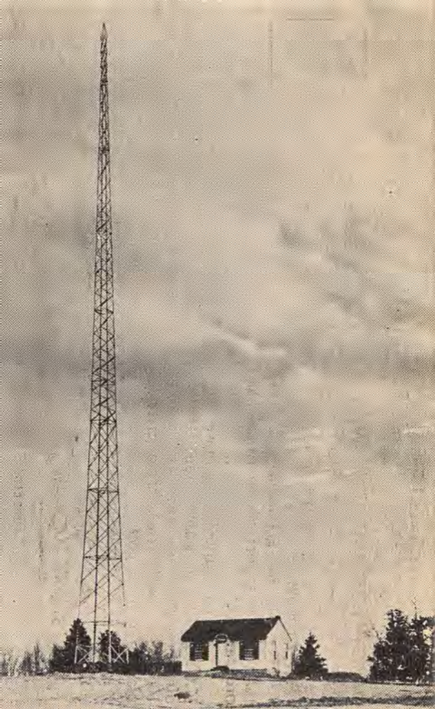
C H N S Vertical Radiating Tower at Bedford, N. S.
