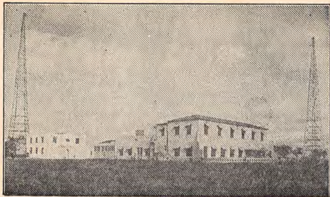
EXTERIOR VIEW XENT. Towers 300 feet, glass insulated, 650 feet apart, 450 feet from building. Licensed for 150,000 watts, now using 100,000 to 75,000 watts.
