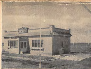
Transmitter Building Middlechurch, Man.
