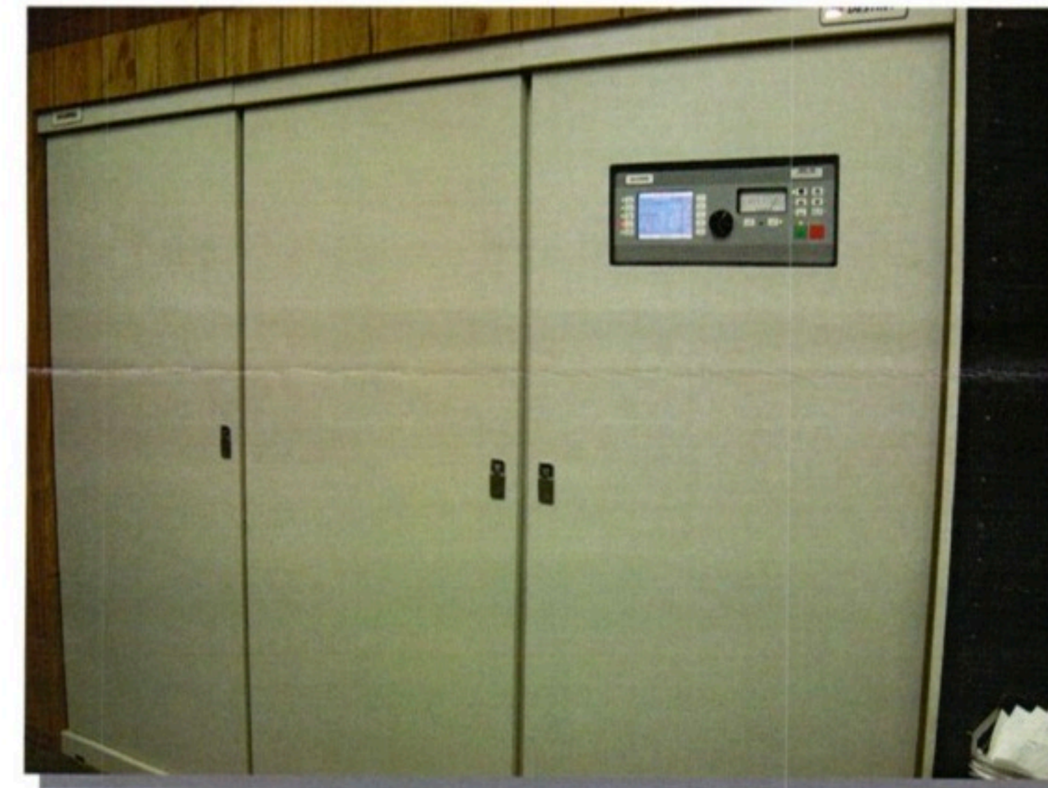
WHK-AM-1220 NEW HARRIS 3DX50 SOLID STATE TRANSMITTER
