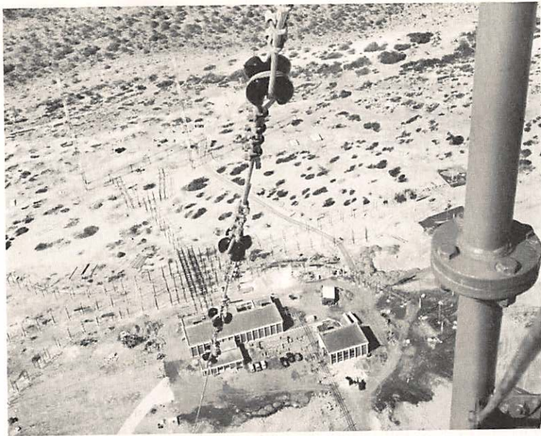
Panoramic view of Trans World Radio's transmitter and diesel generator buildings flanked by the short wave antenna fields, as seen from the top of the 760 foot (233 meters) medium wave antenna.
