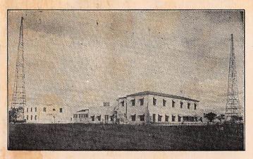
EXTERIOR VIEW XENT. Towers 300 feet, glass insulated, 650 feet apart, 450 feet from building. Licensed for 150,000 watts, now using 100,000 to 75,000 watts.
