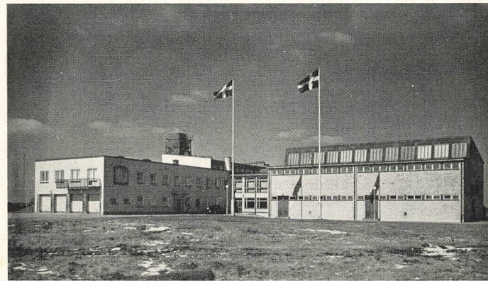
Radio Sweden's powerful 100 kW short-wave transmitters are situated at Hörby, on the plains of Skåne, South Sweden.
