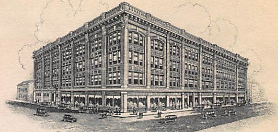
ELEVENTH AVENUE BUILDING
