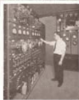
Left, the large Control Panel and Radio Engineer
