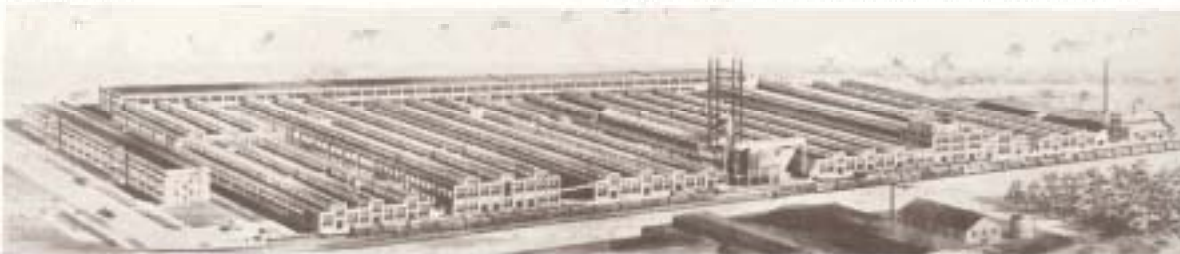
Aerial view of the Willard plant where 10,000 batteries are produced daily
