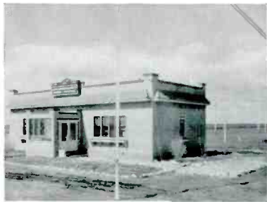
Transmitter Building Middlechurch, Man.
