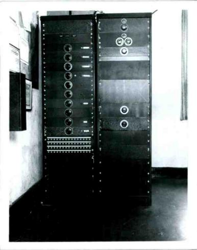
Speech Amplifier Relay Rack and intercom circuits.
