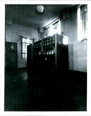
Main Transmitter & Auxillary 500 Watts Output.
