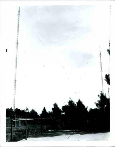
Antenna system, with leflector, 2490 K.C., located Fire Control Station Balboa Park.
