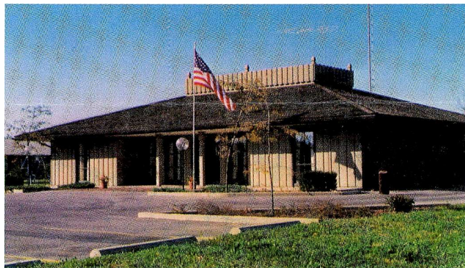
LIMA BROADCAST HOUSE 1301 N. CABLE ROAD, LIMA, OHIO HOME OF RADIO STATIONS WCIT-WLSR
