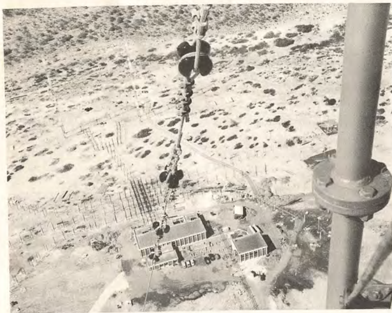
Panoramic view of Trans World Radio's transmitter and diesel generator buildings flanked by the short wave antenna fields, as seen from the top of the 760 foot (233 meters) medium wave antenna.
