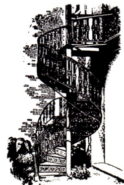
REAR ENTRANCE KNOC
