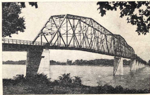
Traffic Bridge Over Mississippi River at Cape Girardeau, Mo.
