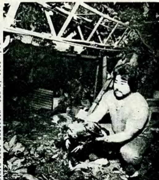
TOWER COLLAPSE—At least six of James Miyashiro's chickens were killed when KDEO's transmitting tower came crashing through his avocado trees last night. The tower missed Miyashiro's house by about 15 feet. —Star-Bulletin Photo by Dean Sensui.
